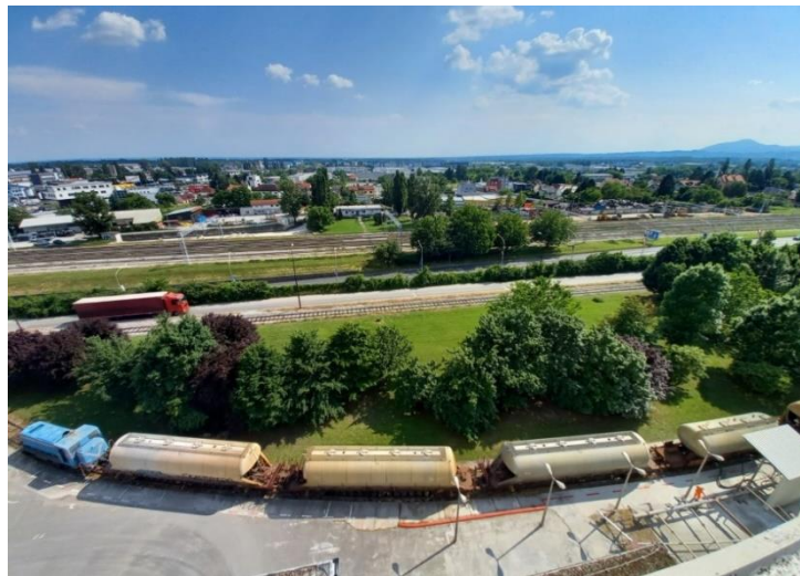
Figure 5. Terminal Podsused location (Source: CEMEX Croatia, 2022)
