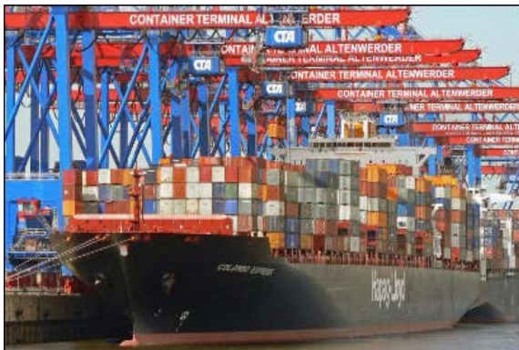
Figure 1. Port container terminal
